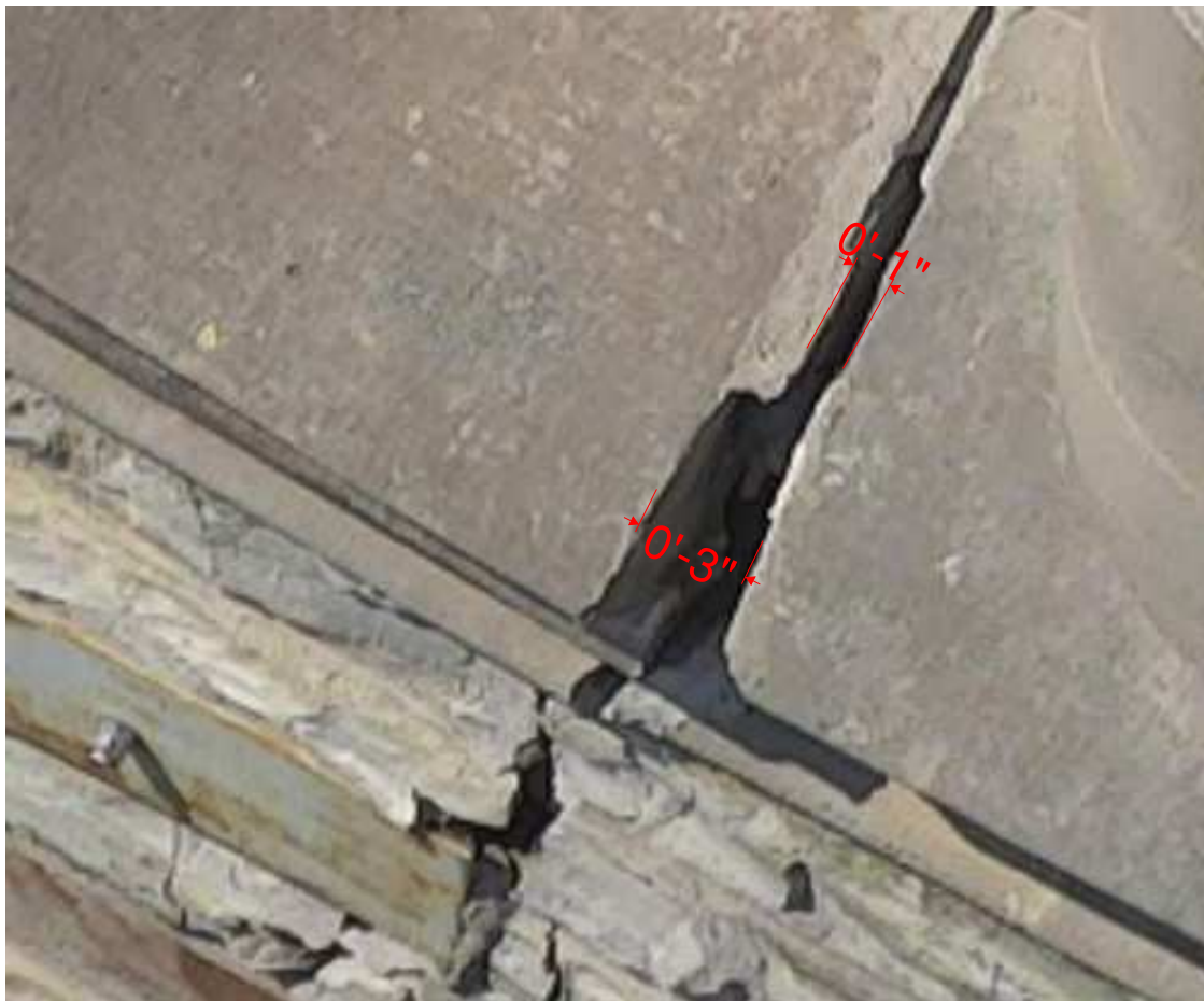
Figure 7: Comparison of Cracks at East face of Tower
