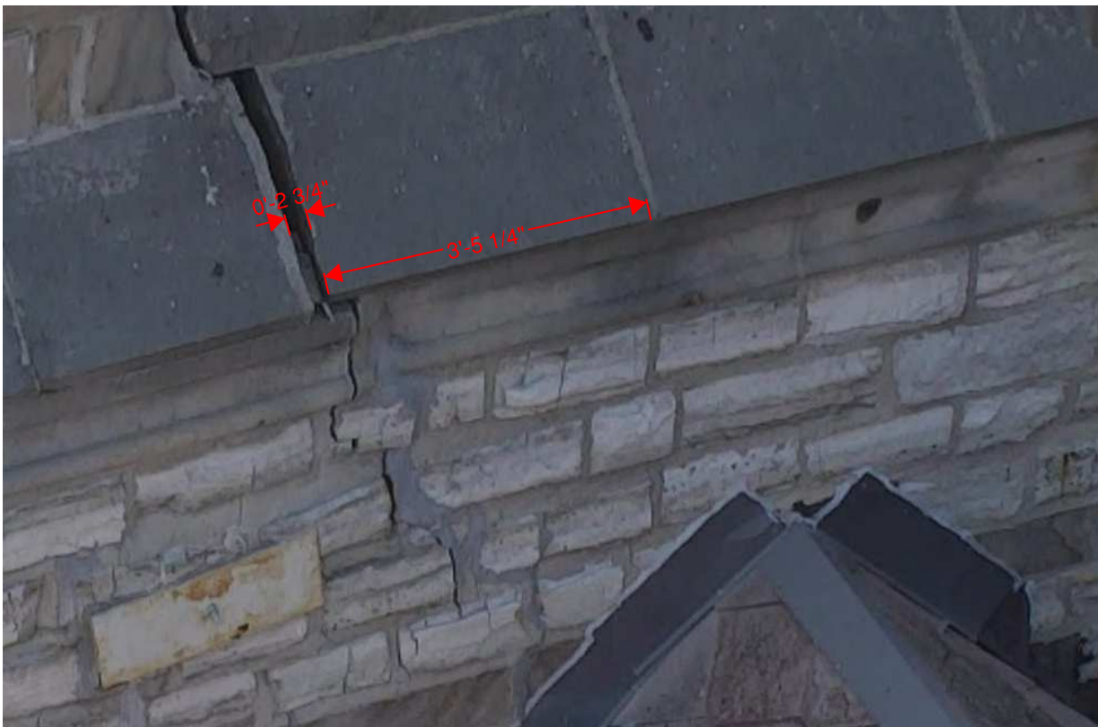
Figure 8: Crack at North Side of Tower
