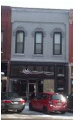
225 Central Avenue - Palisades
