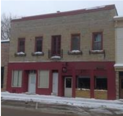
116 Central Avenue (114 & 116) - Sheesley & Palisades
