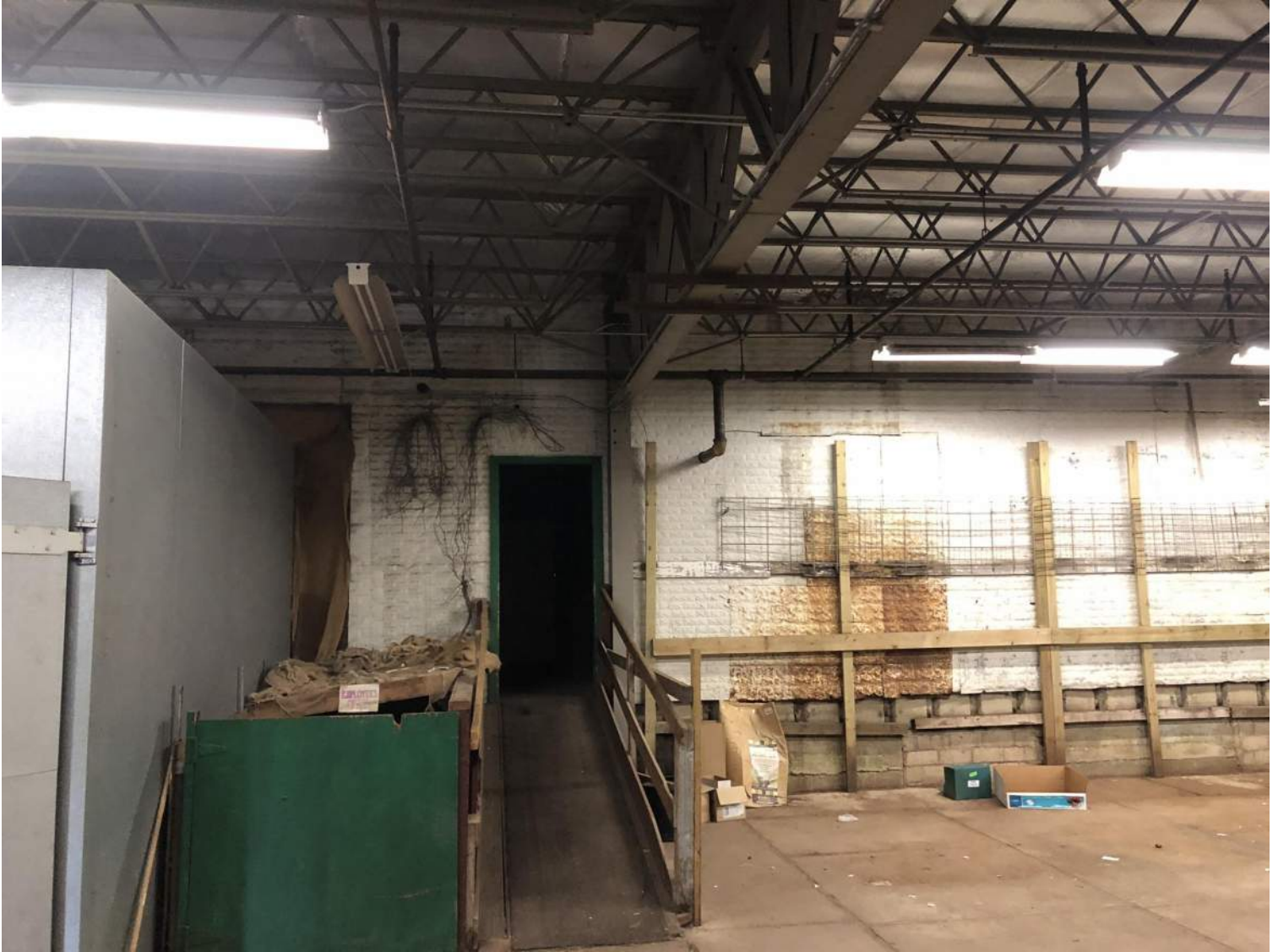
FIGURE 10 - TYPICAL STEEL FRAMING SEEN WITHIN THE STEEL-FRAMED BUILDING (CIRCA 1930).
