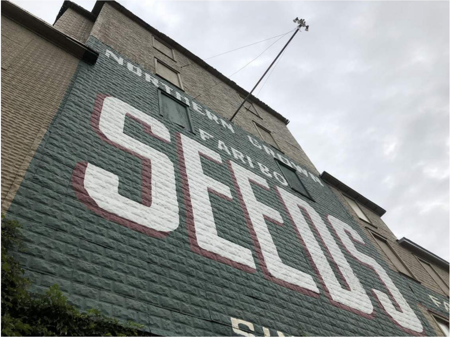
FIGURE 5 - TYPICAL METAL SIDING ON EXTERIOR WALLS. NOTE THE STONE PATTERN STAMPED ON THE METAL SHEETS.
