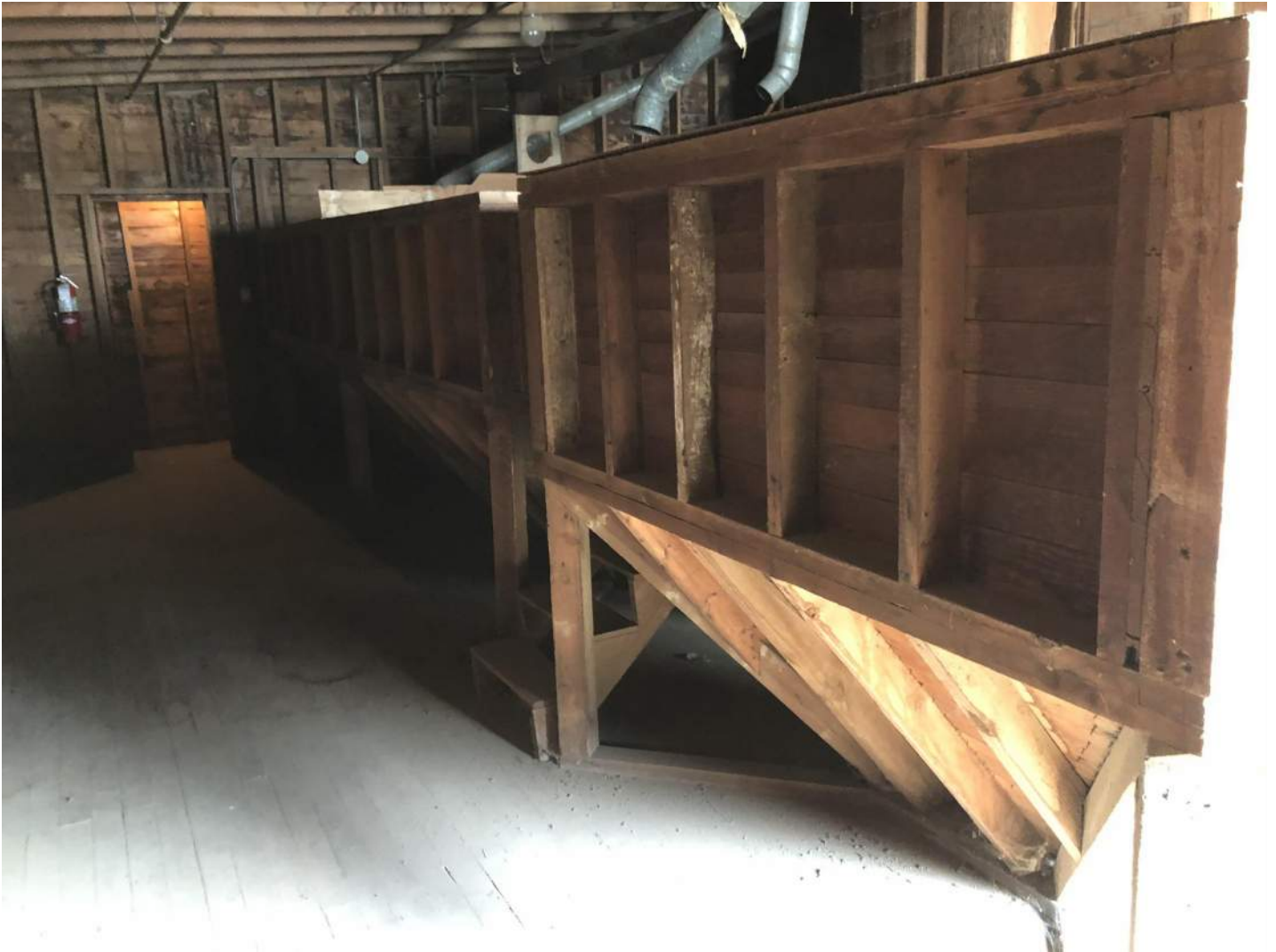
FIGURE 6 - WOODEN HOPPERS USED ON THE UPPER FLOORS OF THE ORIGINAL STRUCTURE.
