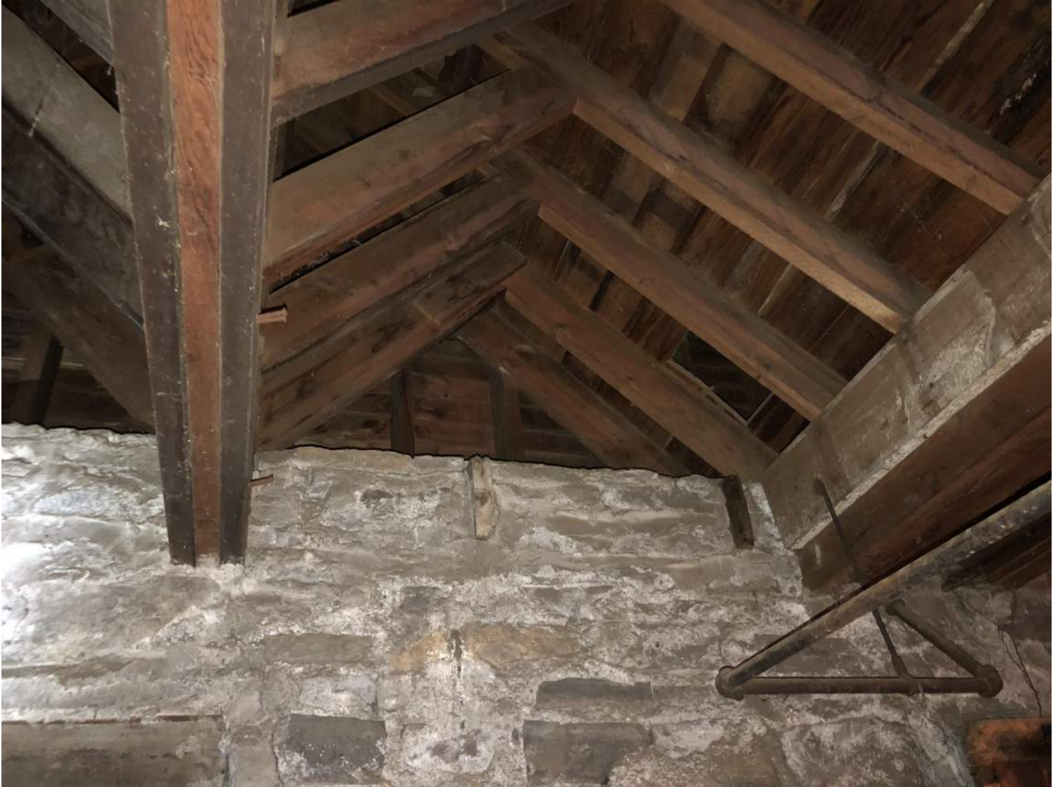
FIGURE 8 - TYPICAL WOOD FRAMING AT THE BASE OF THE MULTI-STORY GRAIN BINS; THIS VIEW IS FROM THE FIRST FLOOR OF THE BUILDING. THE ROCK-FACED FARIBAULT STONE CAN BE SEEN SUPPORTING THE WOOD FRAMING OF THE GRAIN BINS.
