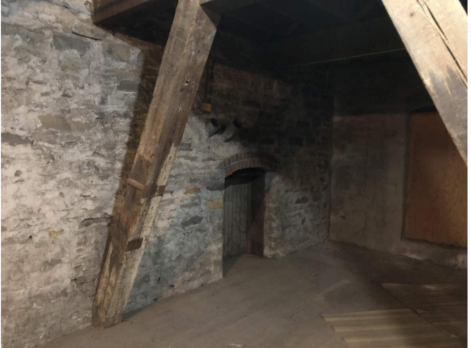
FIGURE 9 - TYPICAL WOOD FRAMING AND BRACING ADJACENT TO A STONE WALL ON THE LOWER FLOORS OF THE MAIN WOOD BUILDING. .
