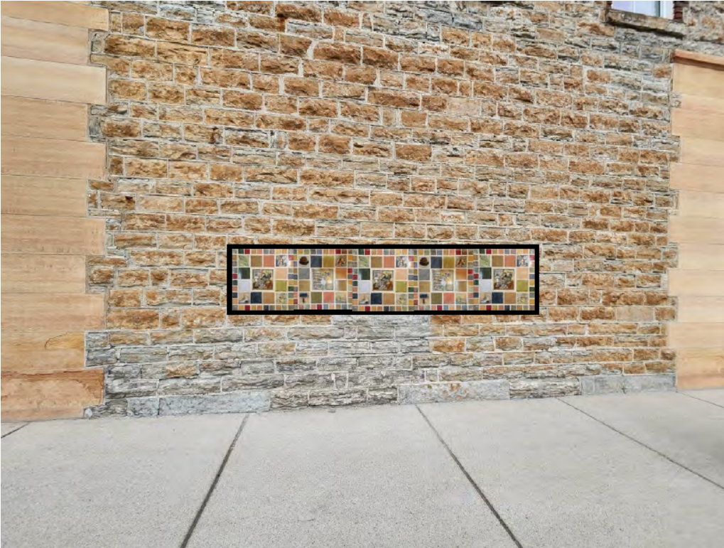
South Wall of 301 Central Avenue
