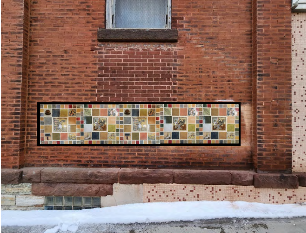
North Wall of 329 Central Avenue
