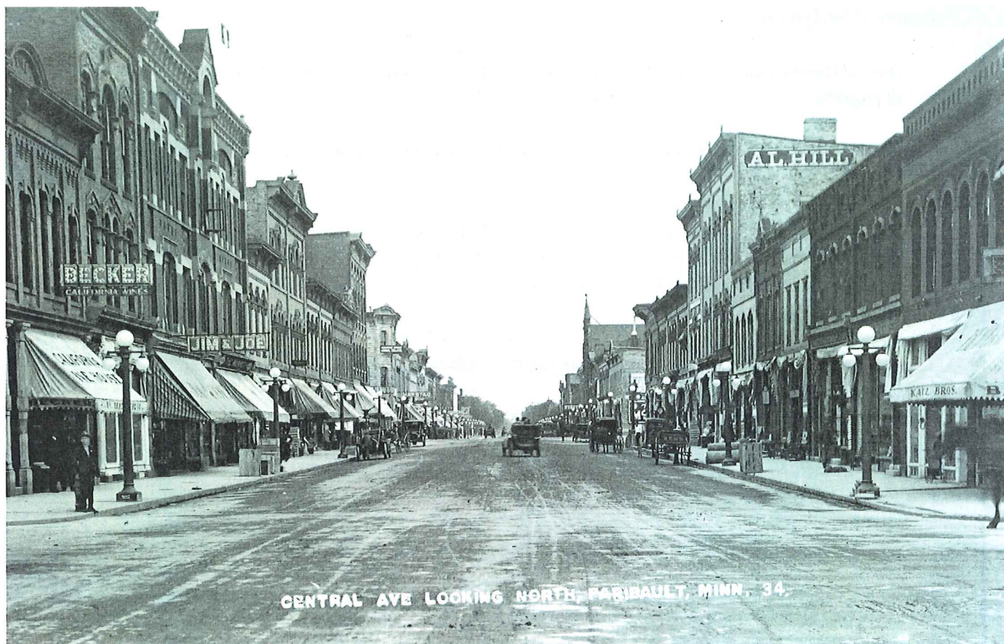
Photograph taken ca 1910, looking north at the 200 block of Central Avenue.
