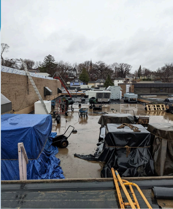
Roof & HVAC Replacement
