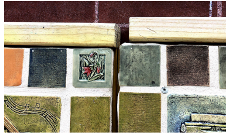
Installed Tile Frame at 329 Central
