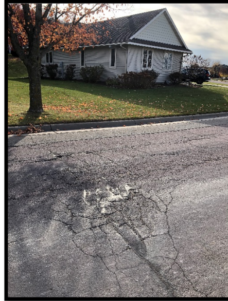
Newhall Drive Pavement Examples
