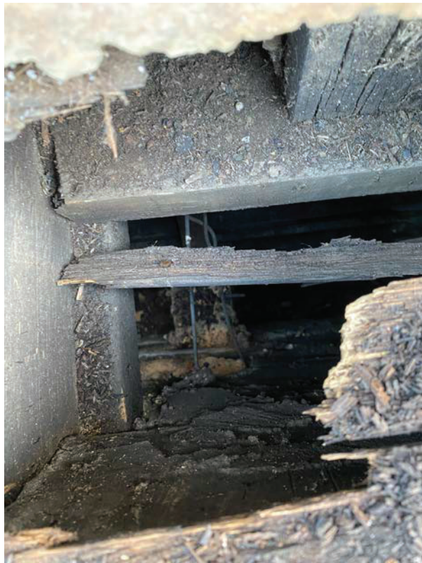
Picture 4: Existing rotted parapet and overhang framing.
