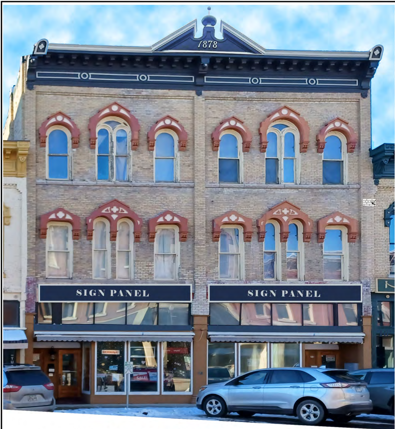
Replacement of Historic Sign Panels - colors to match new Building Cornice
