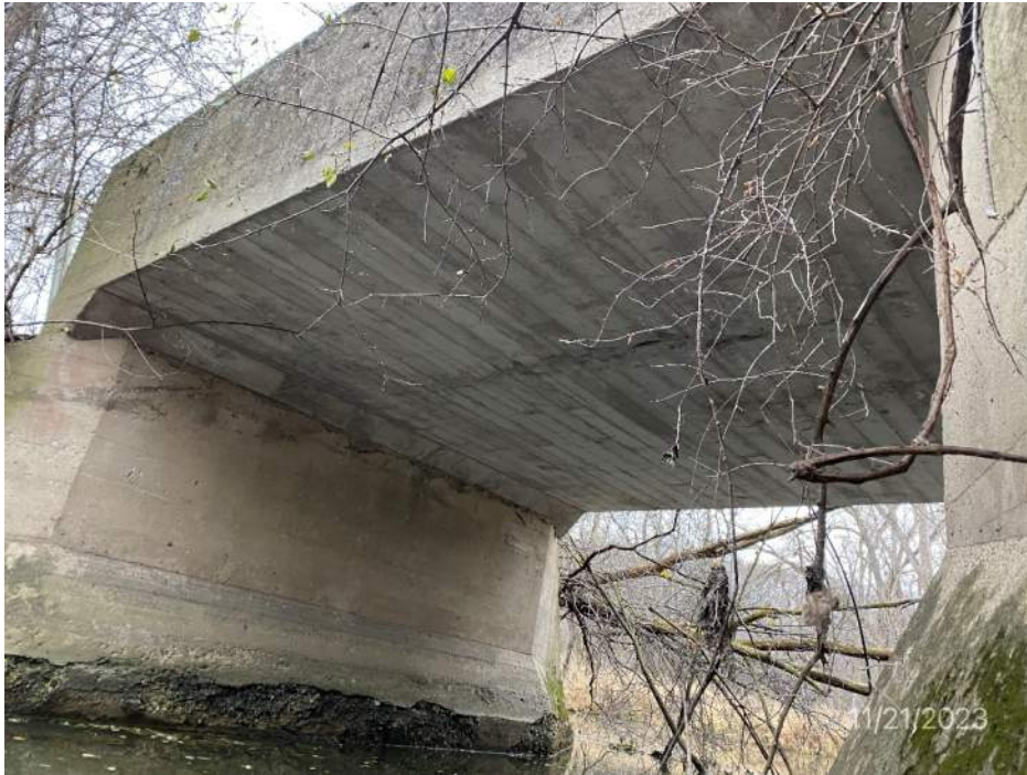
Concrete culvert looking southwest
