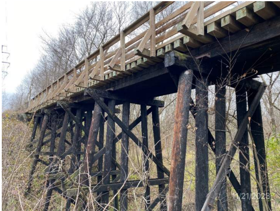
Pier 5 looking southwest
