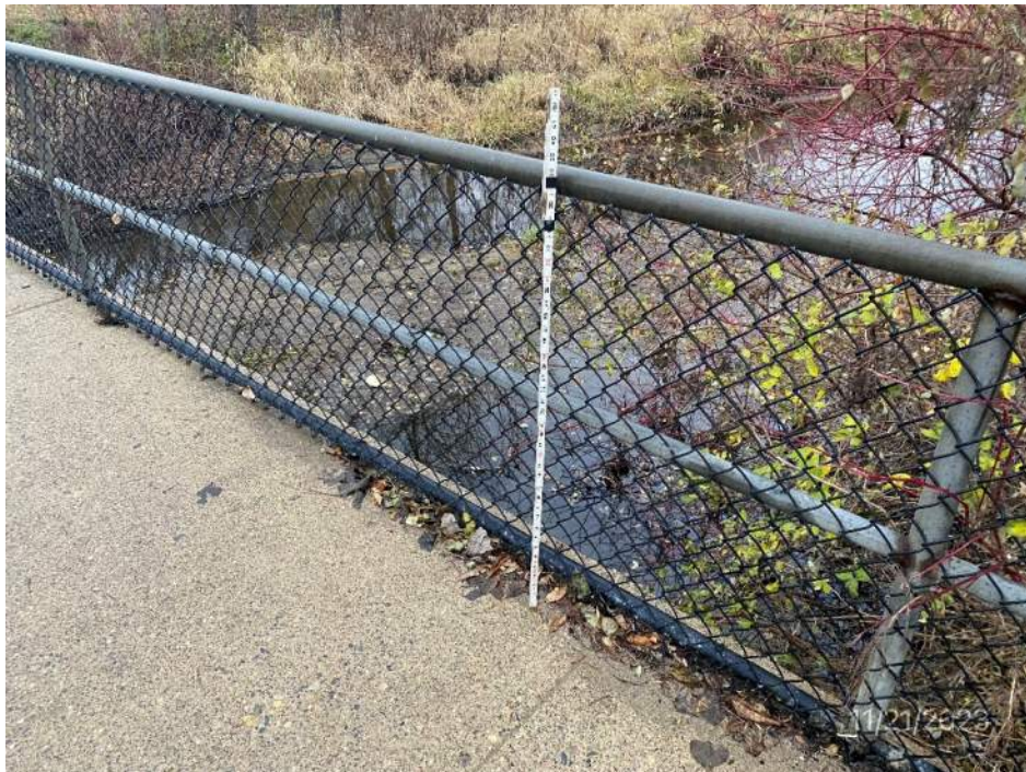
Bridge rail looking southeast
