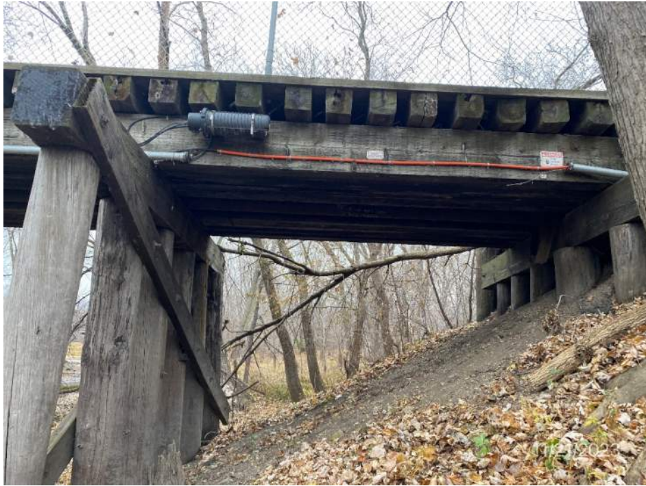
Span 1 looking east with High-Voltage Utility line
