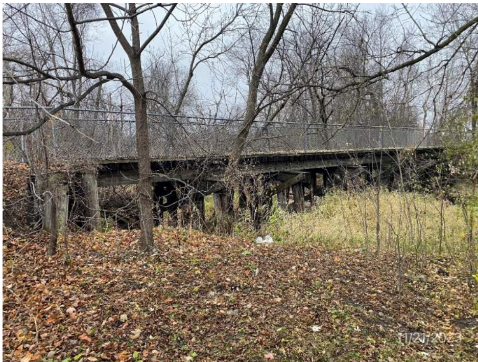
General elevation looking north
