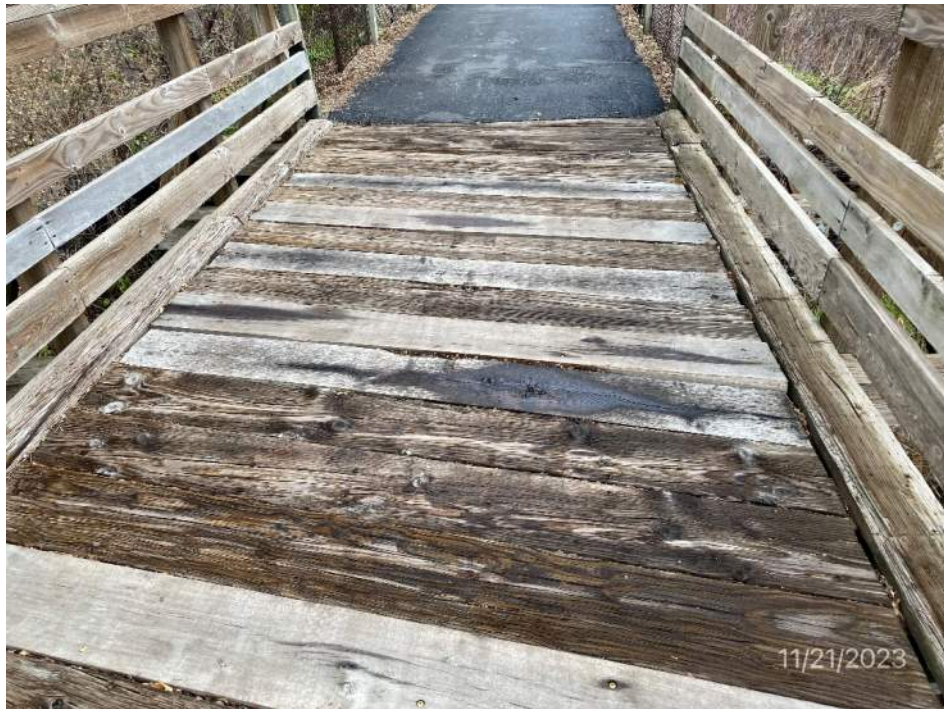
Timber deck near south approach
