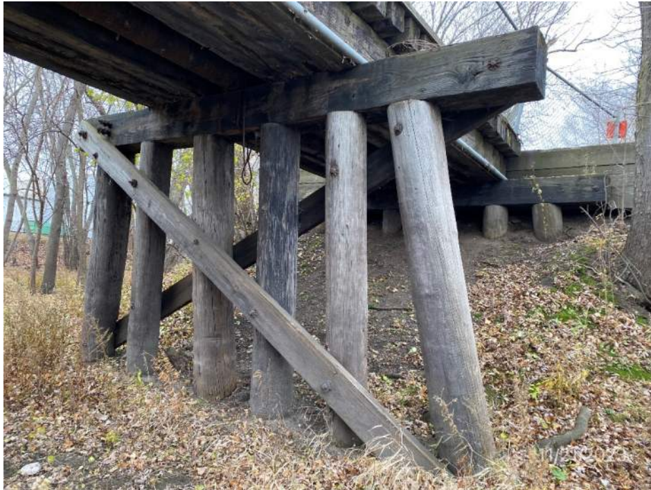
Pier 1 looking southeast
