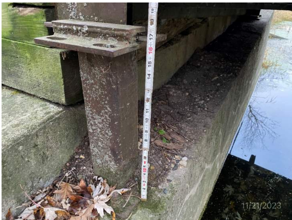
Bearing at southeast abutment corner
