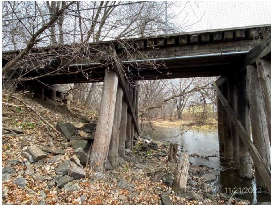
Piers 7 and 8 looking east
