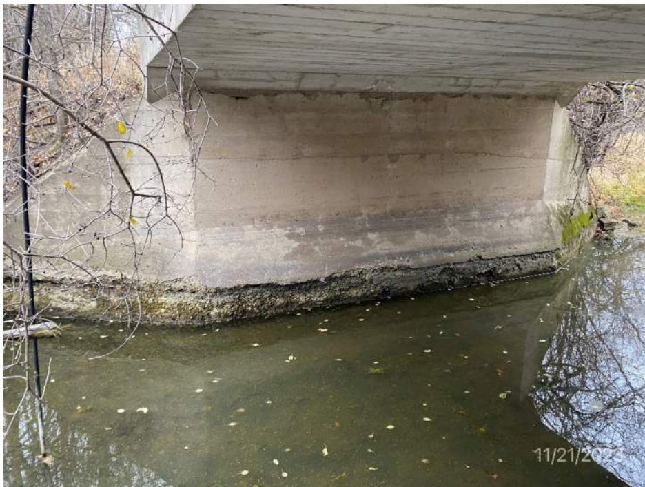
North culvert wall
