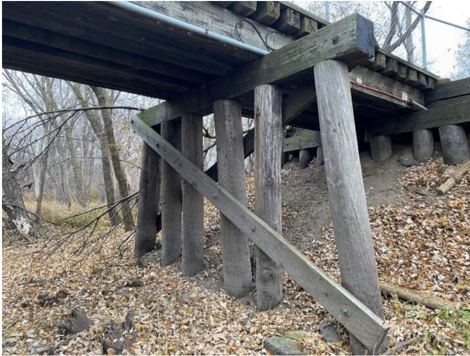
Pier 1 looking southeast
