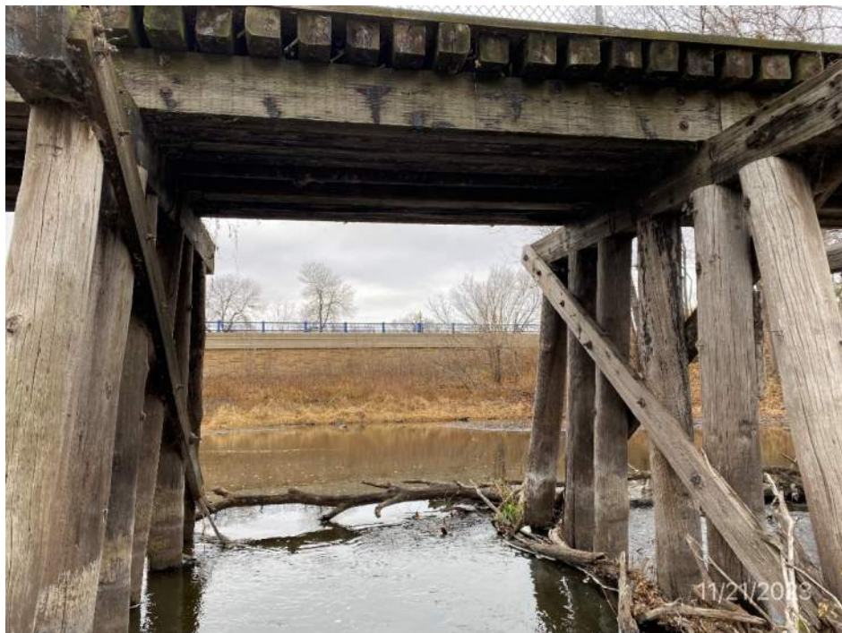
Span 4 and Pier 4 looking west
