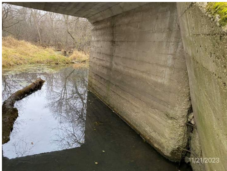
South culvert wall
