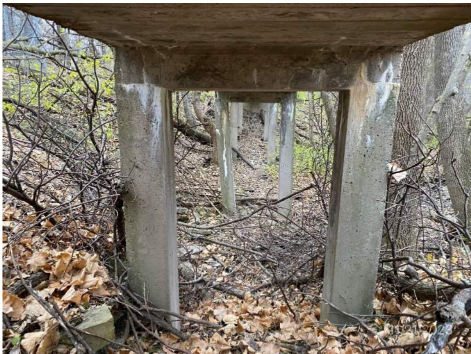
Pier 1 looking east
