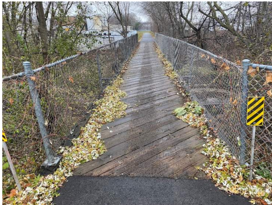
Sakatah Trail and bridge deck looking west
