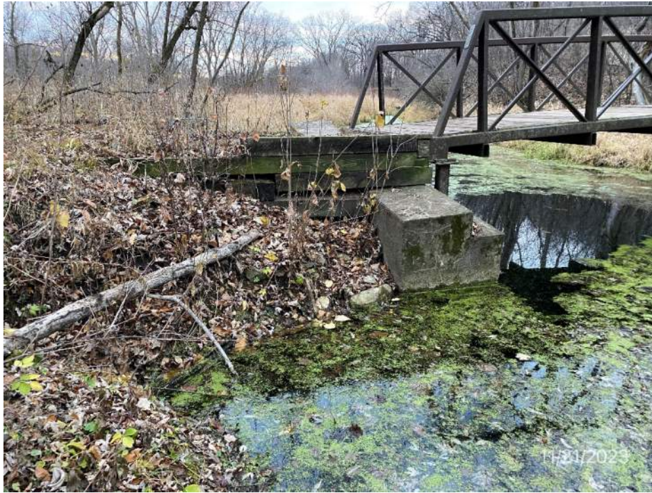
Timber retaining wall at southeast corner
