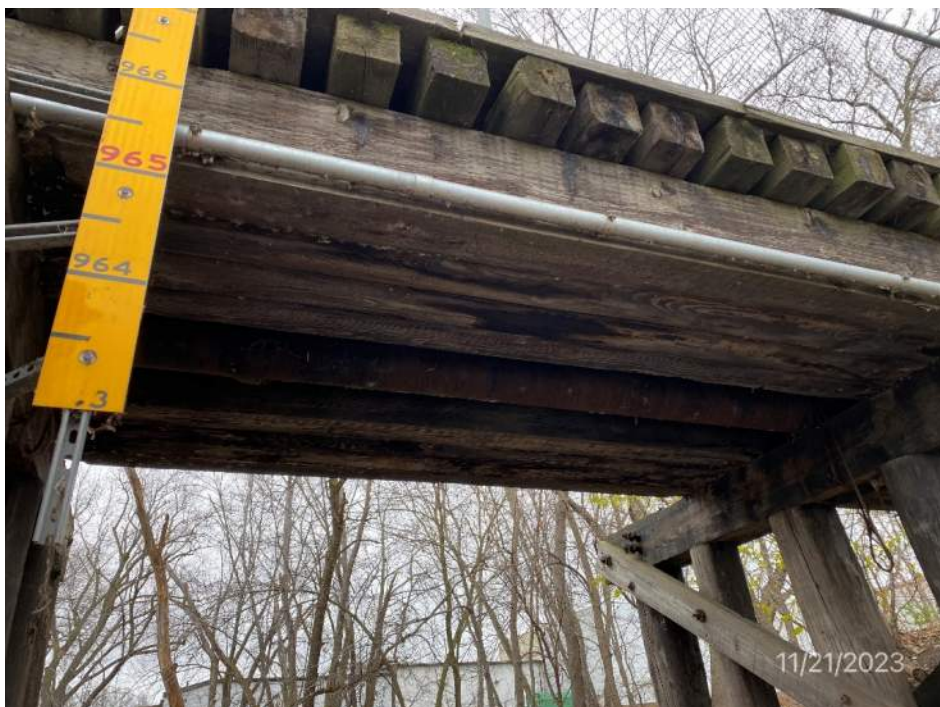
Span 2 superstructure looking east with High-Voltage Utility line
