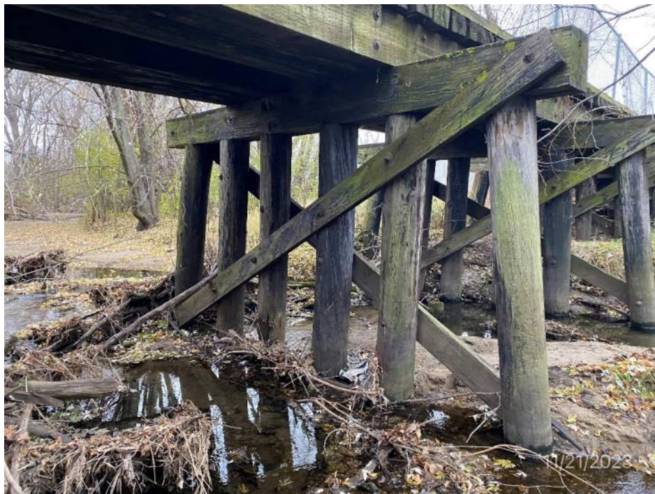
Pier 3 looking southwest
