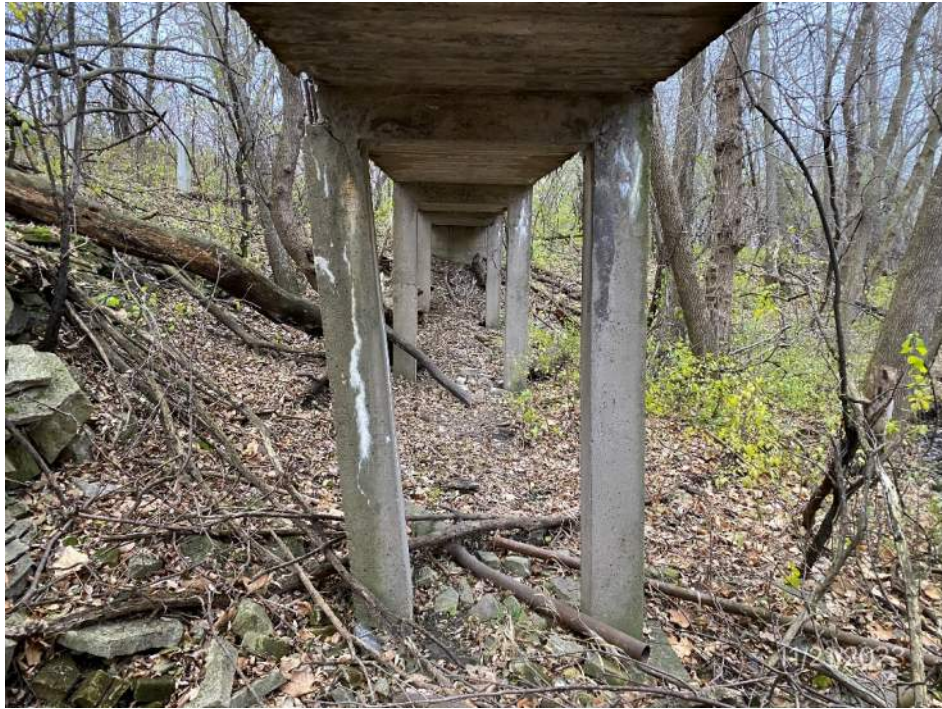
Pier 2 looking east
