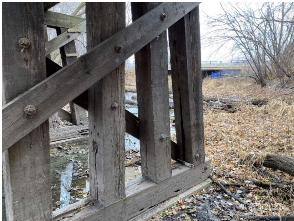
Pier 4 looking southwest
