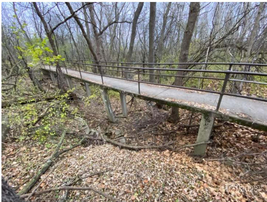
General elevation looking southeast
