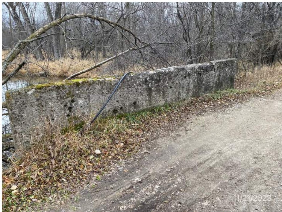
East concrete barrier
