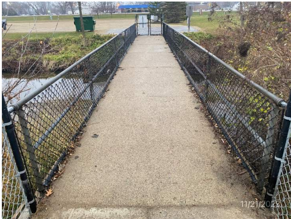
Bridge deck looking east
