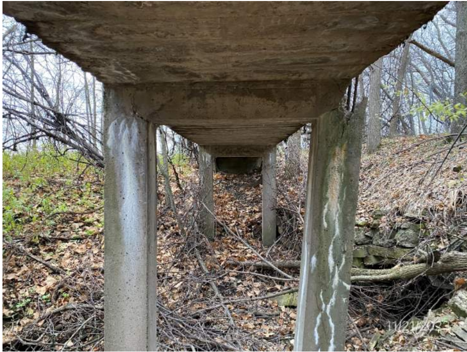
Pier 2 looking west
