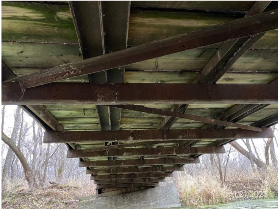
General superstructure looking south
