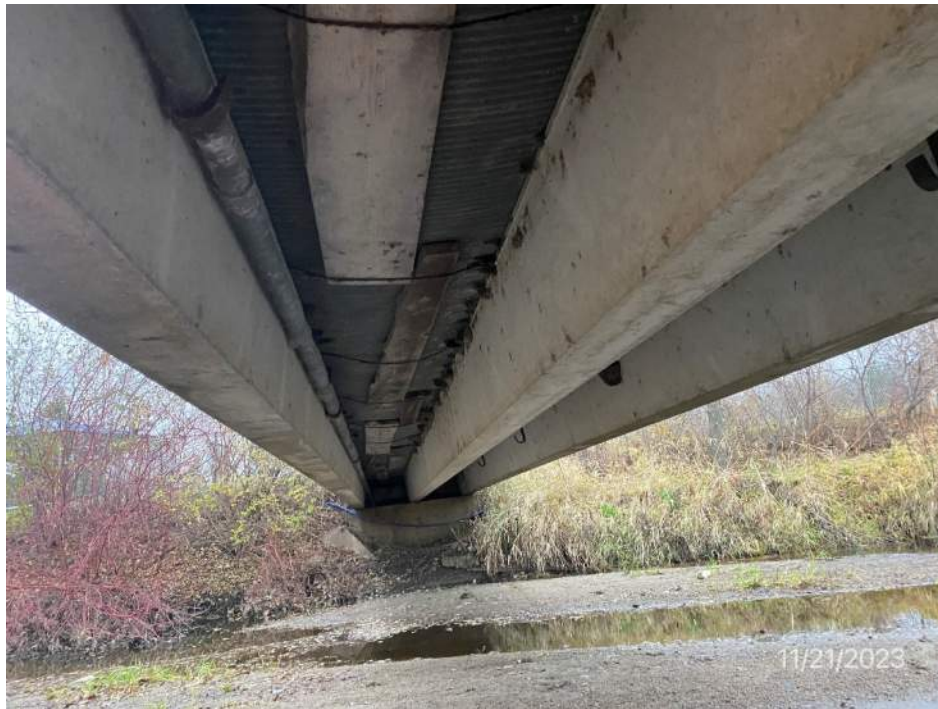
General superstructure looking west
