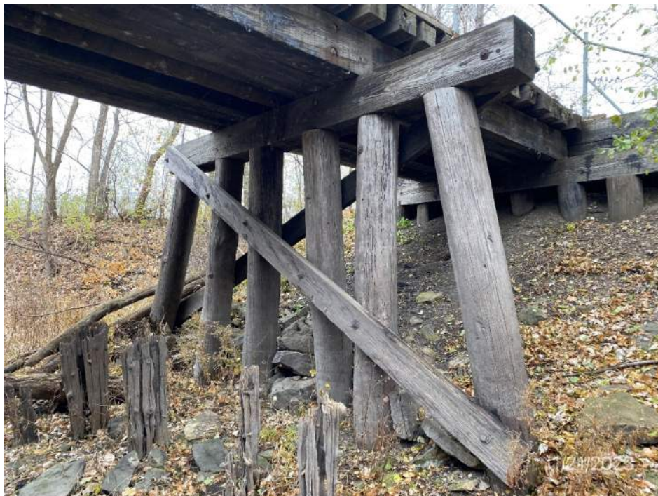
Pier 5 looking northwest
