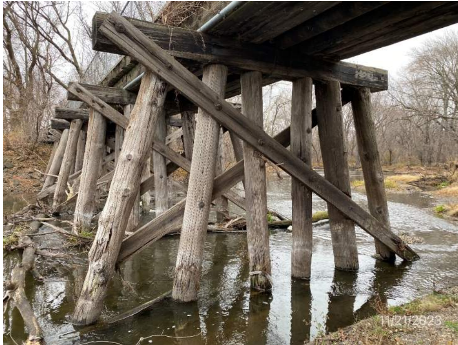
Pier 3 looking north
