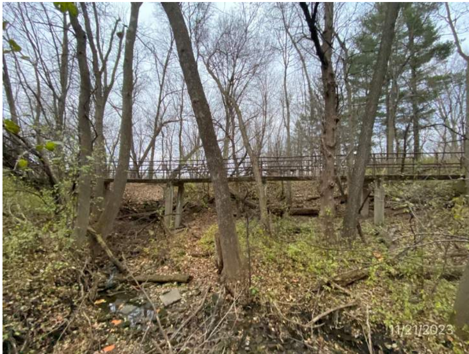
General elevation looking north
