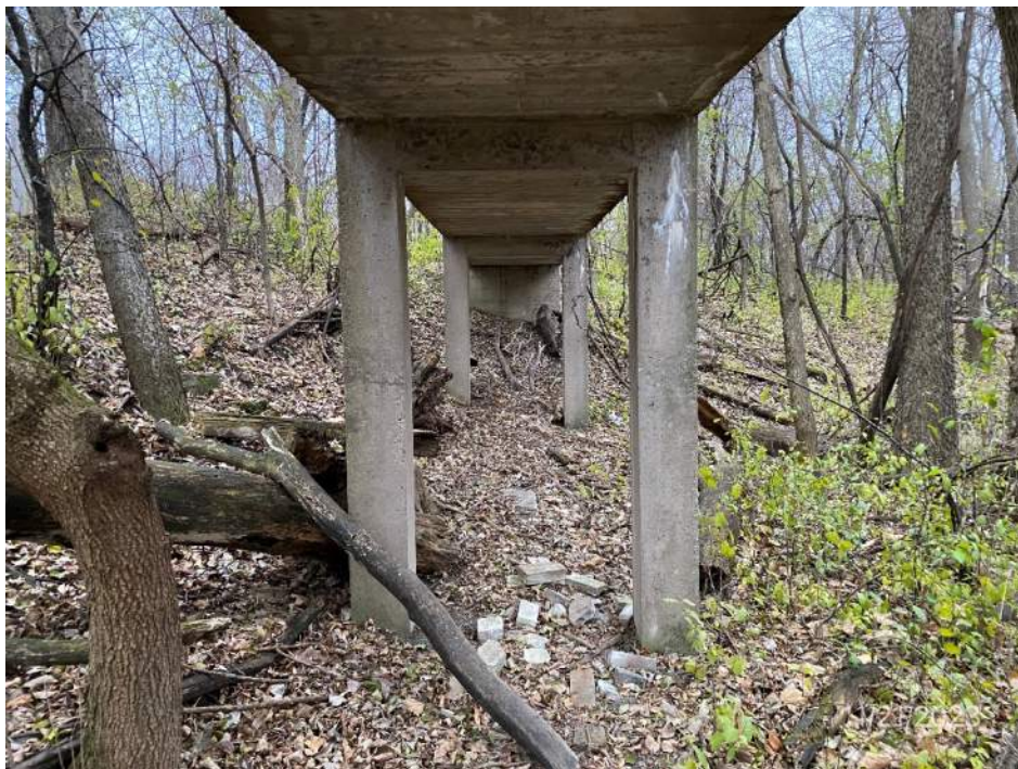
Pier 3 looking east
