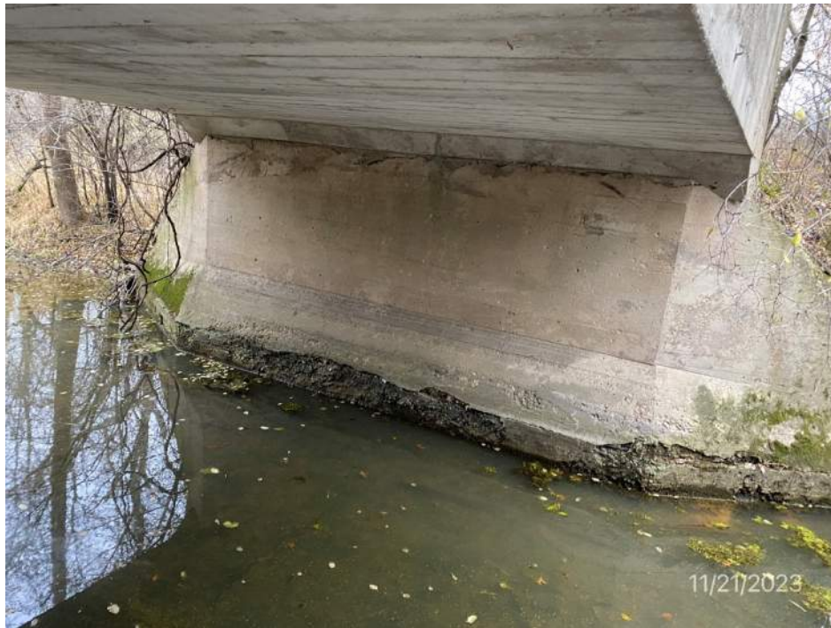
South culvert wall
