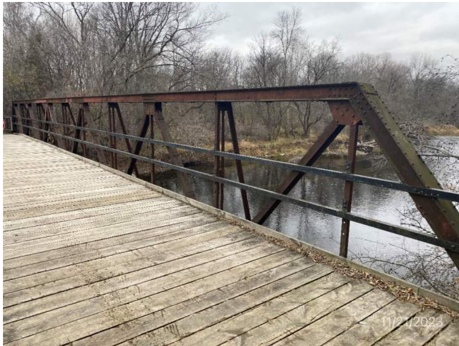
Timber deck and steel rail looking southwest
