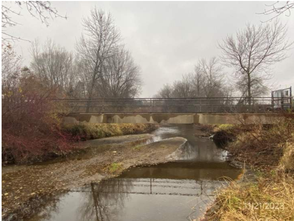
General elevation looking north
