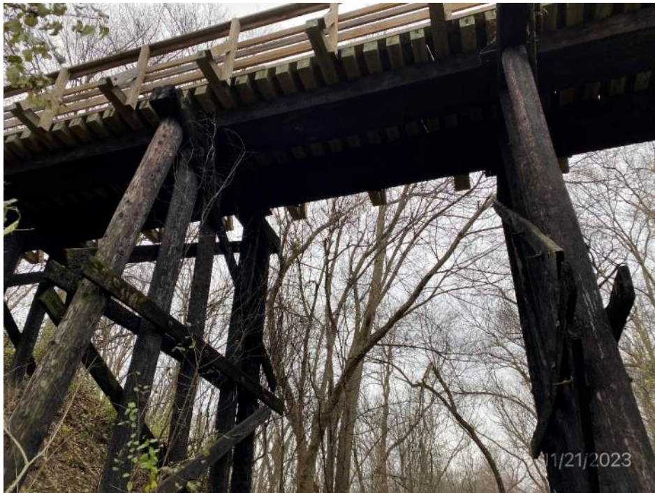
Piers 2 and 3 looking west
