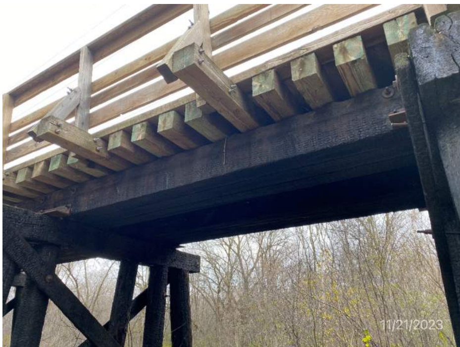
Span 2 superstructure looking east
