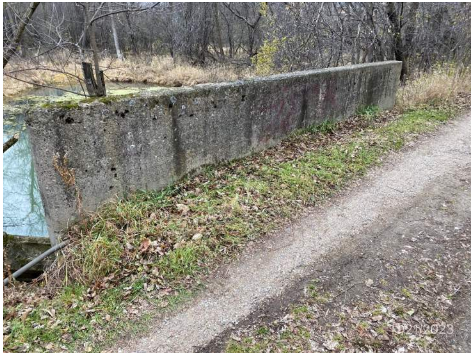
East concrete barrier
