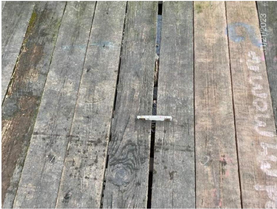
General condition of timber deck
