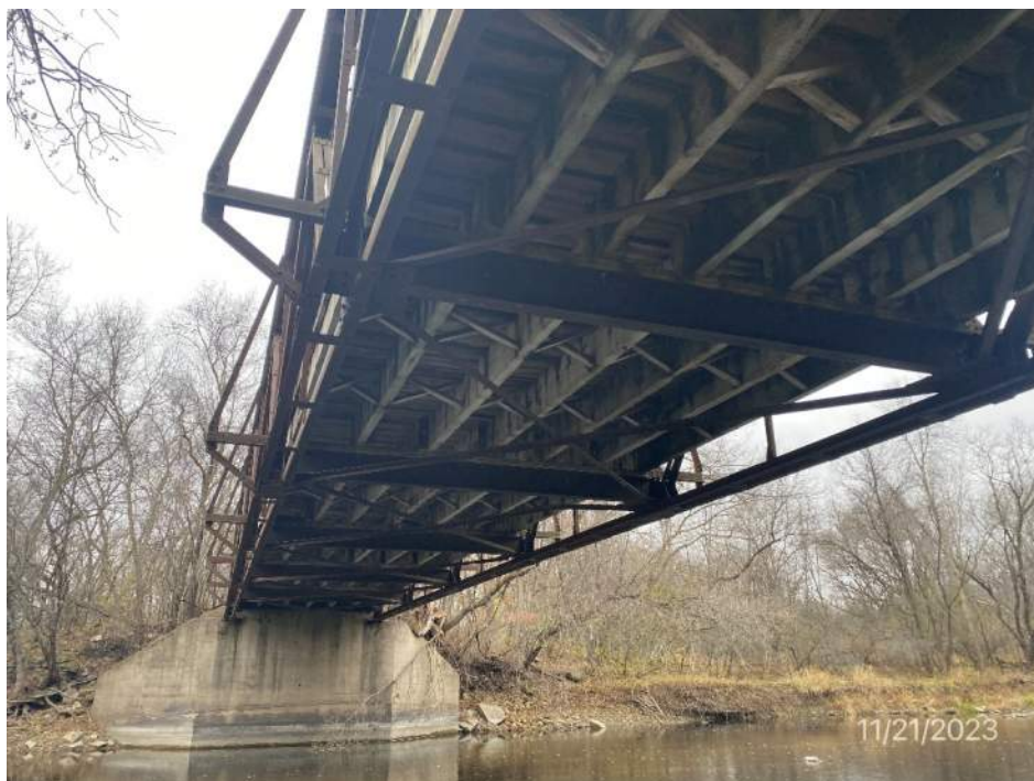
North Abutment and General Superstructure looking north
