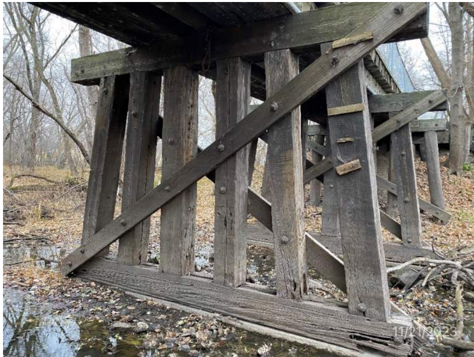
Pier 3 looking south
