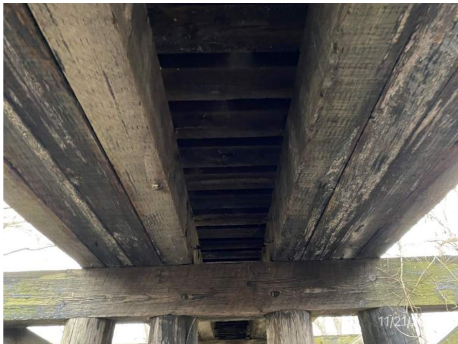
General superstructure, Span 2, looking west
