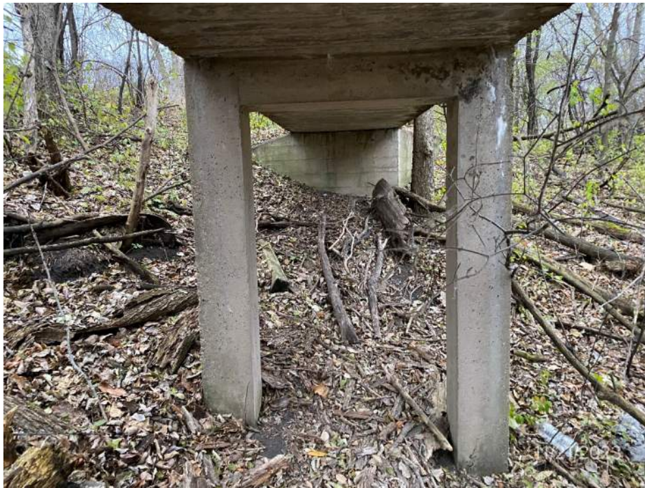
Pier 4 looking east
