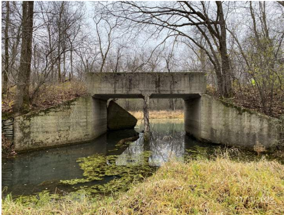
General elevation looking west (unable to photograph elevation looking east due to steep slopes)
