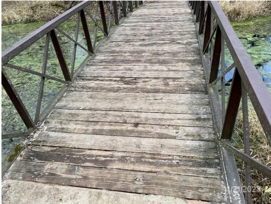
Timber deck looking south
