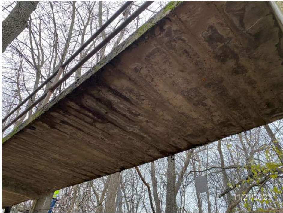
Span 2 superstructure looking northwest, typical at other spans
