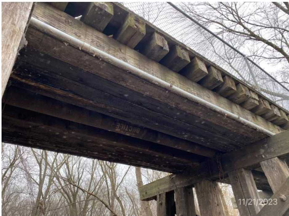
General superstructure at Span 4, looking southeast
