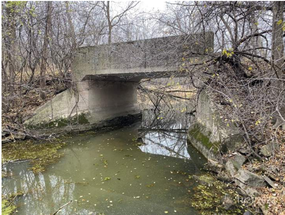
General elevation looking west (unable to take east elevation photo due to steep slopes)
