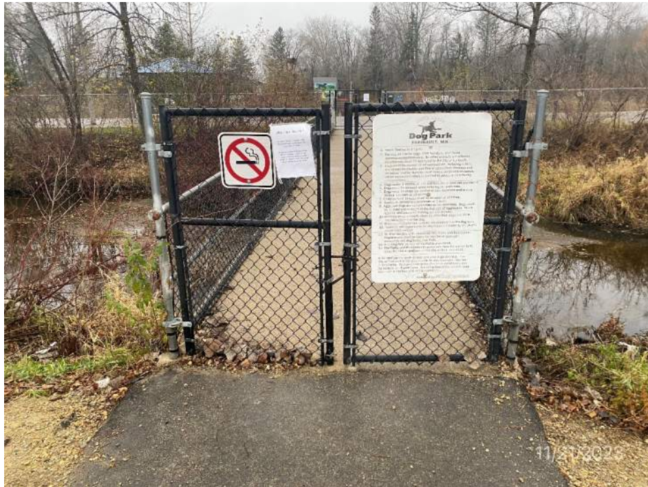
East approach gate, looking west
