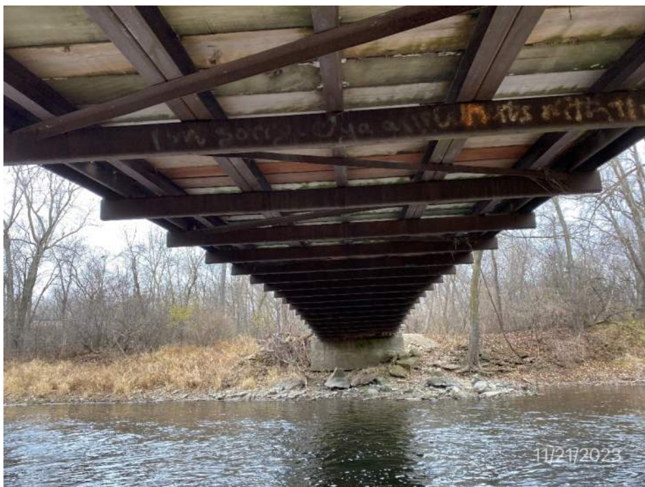
General superstructure looking north
