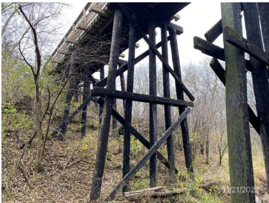
Pier 4 looking north
