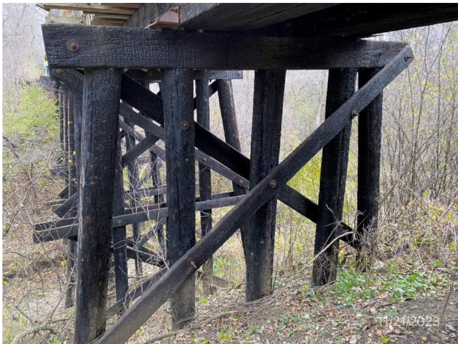
Pier 1 looking north
