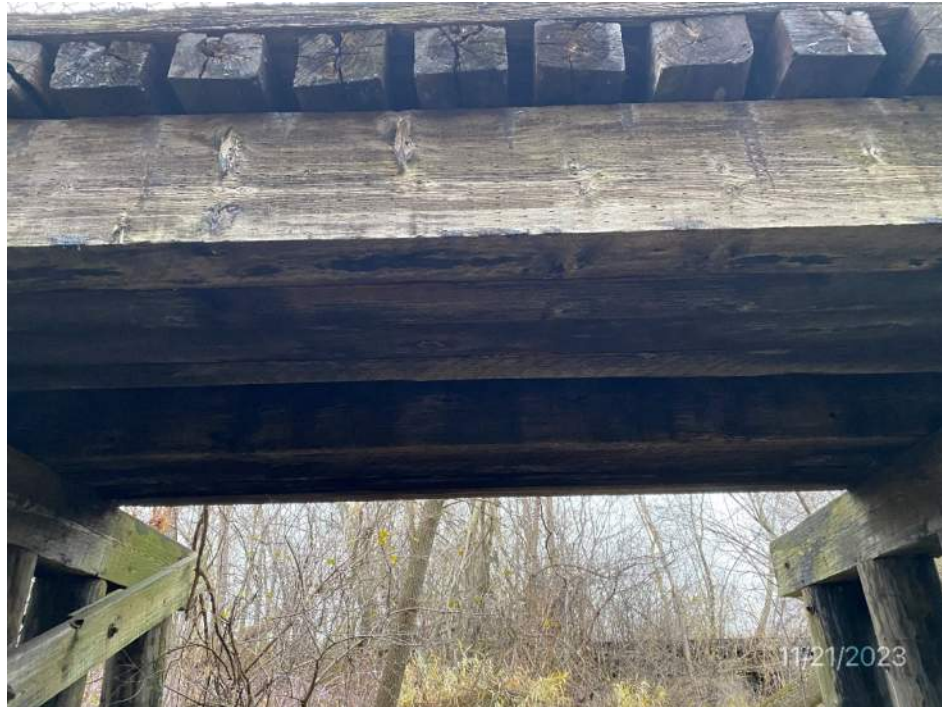
General superstructure, Span 2, looking south
