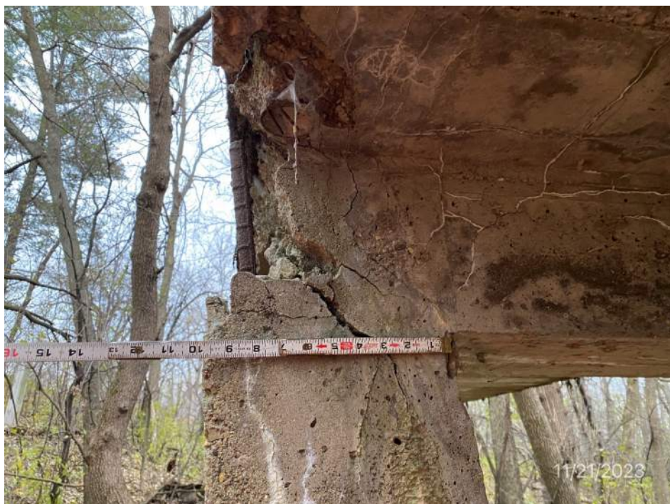
Pier 2, north column looking east
