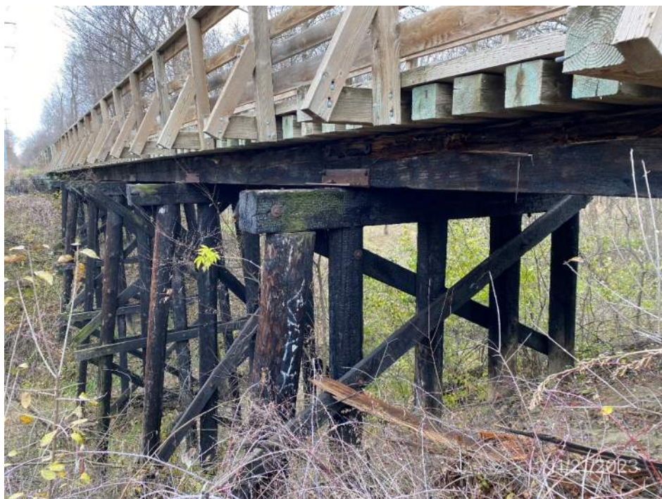
Pier 6 looking southwest
