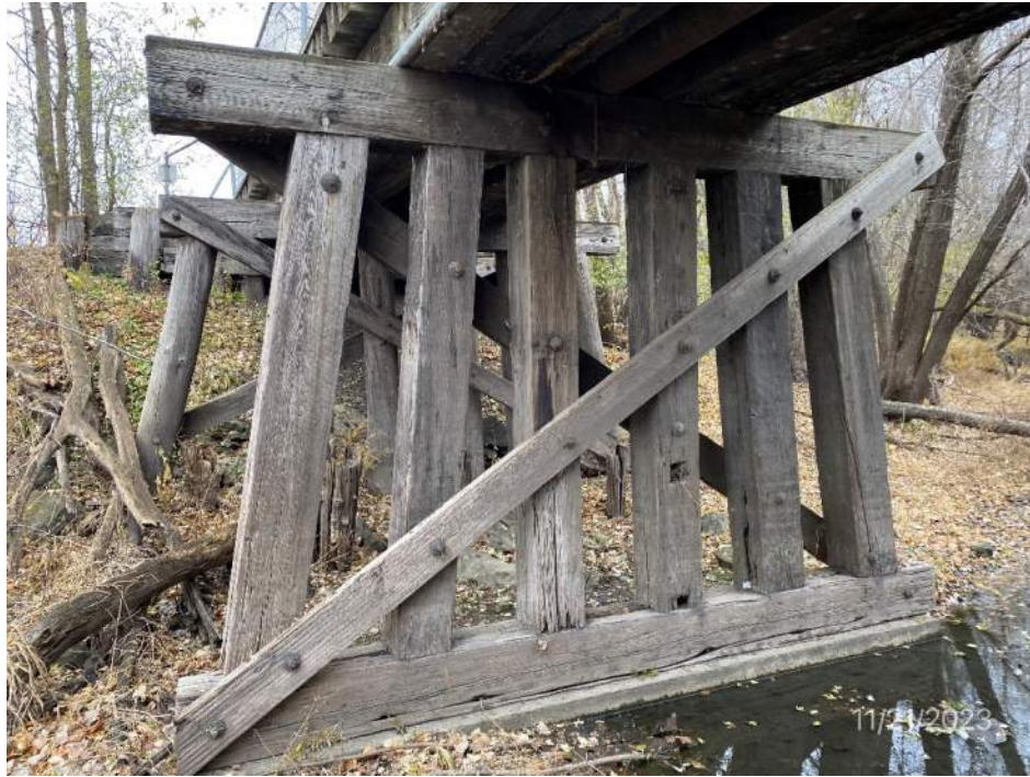
Pier 4 looking north
