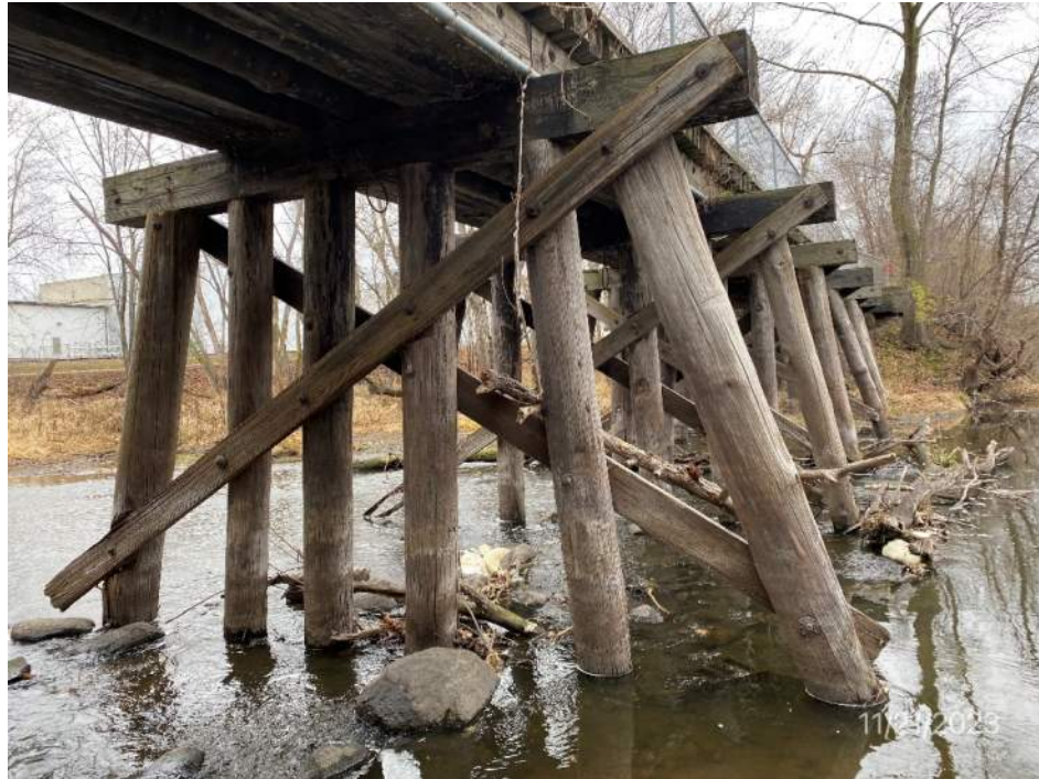
Pier 5 looking south
