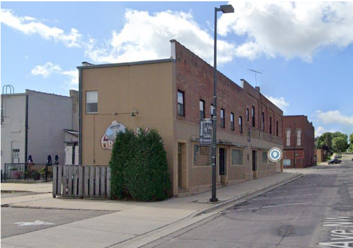
Rear Façade 30 3 rd St. NW (July 2019 Google Earth)
