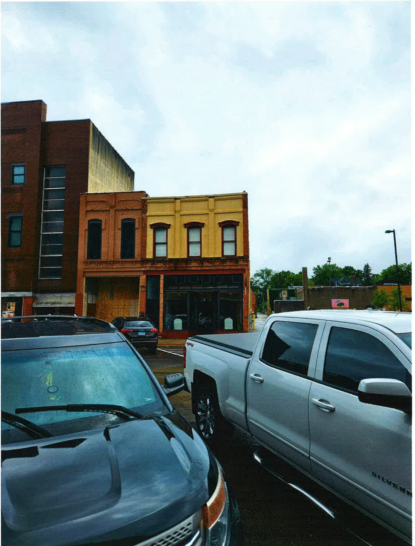
Front of building
