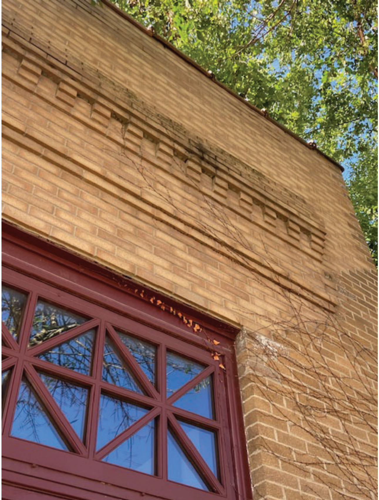
Brick Replacement Complete on NW Corner of Building - Work Approved and Completed in 1993
