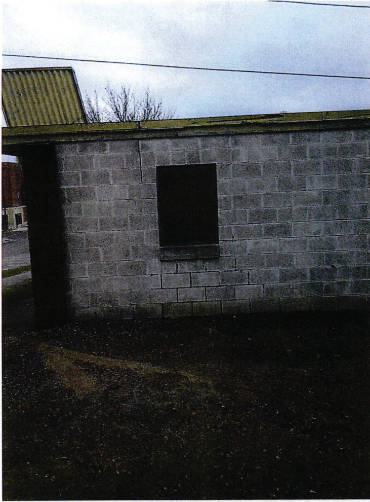
West Side of Building
