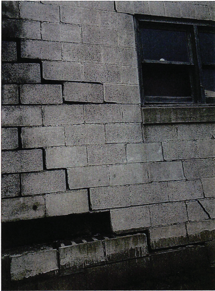
East Side of Building
