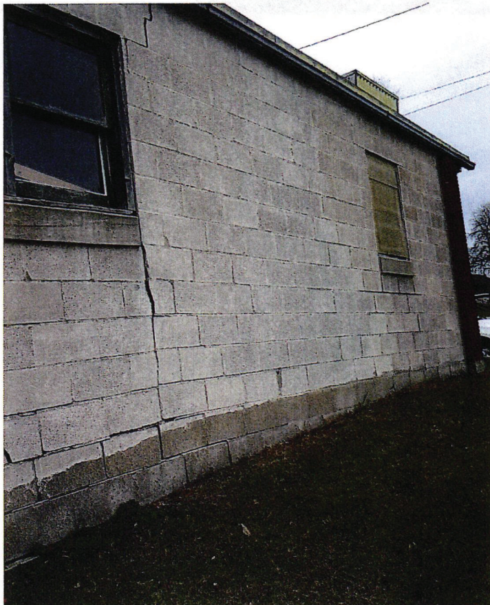
East Side of Building
