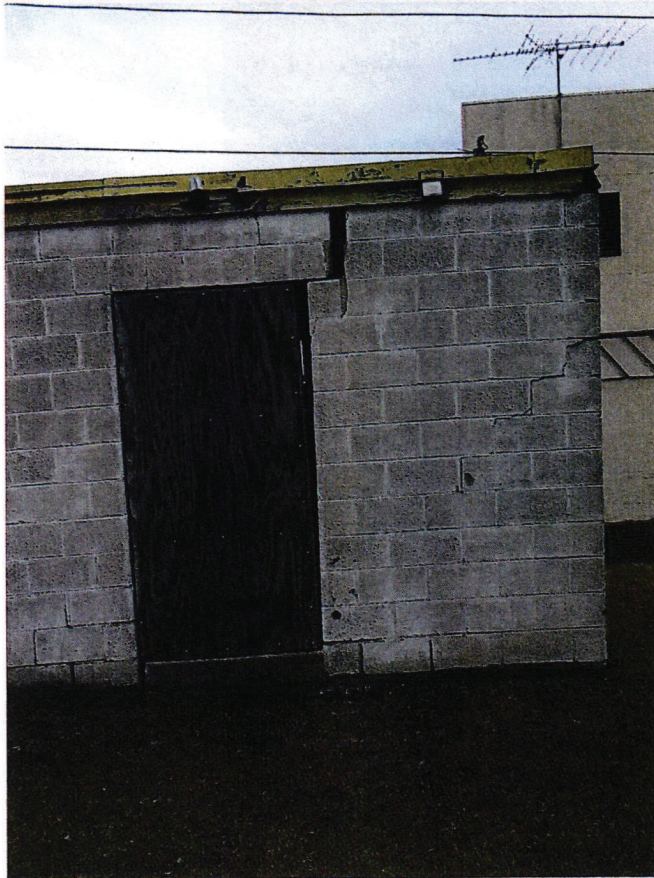
West Side of Building
