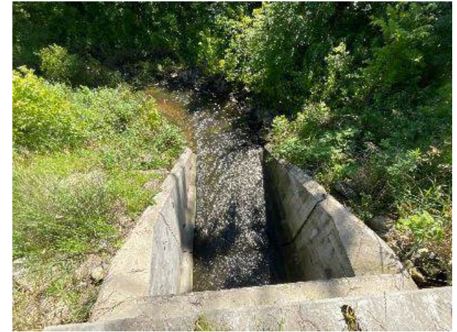
Photo 27: Start of Intermittent Stream 2, flowing east out of culvert.
