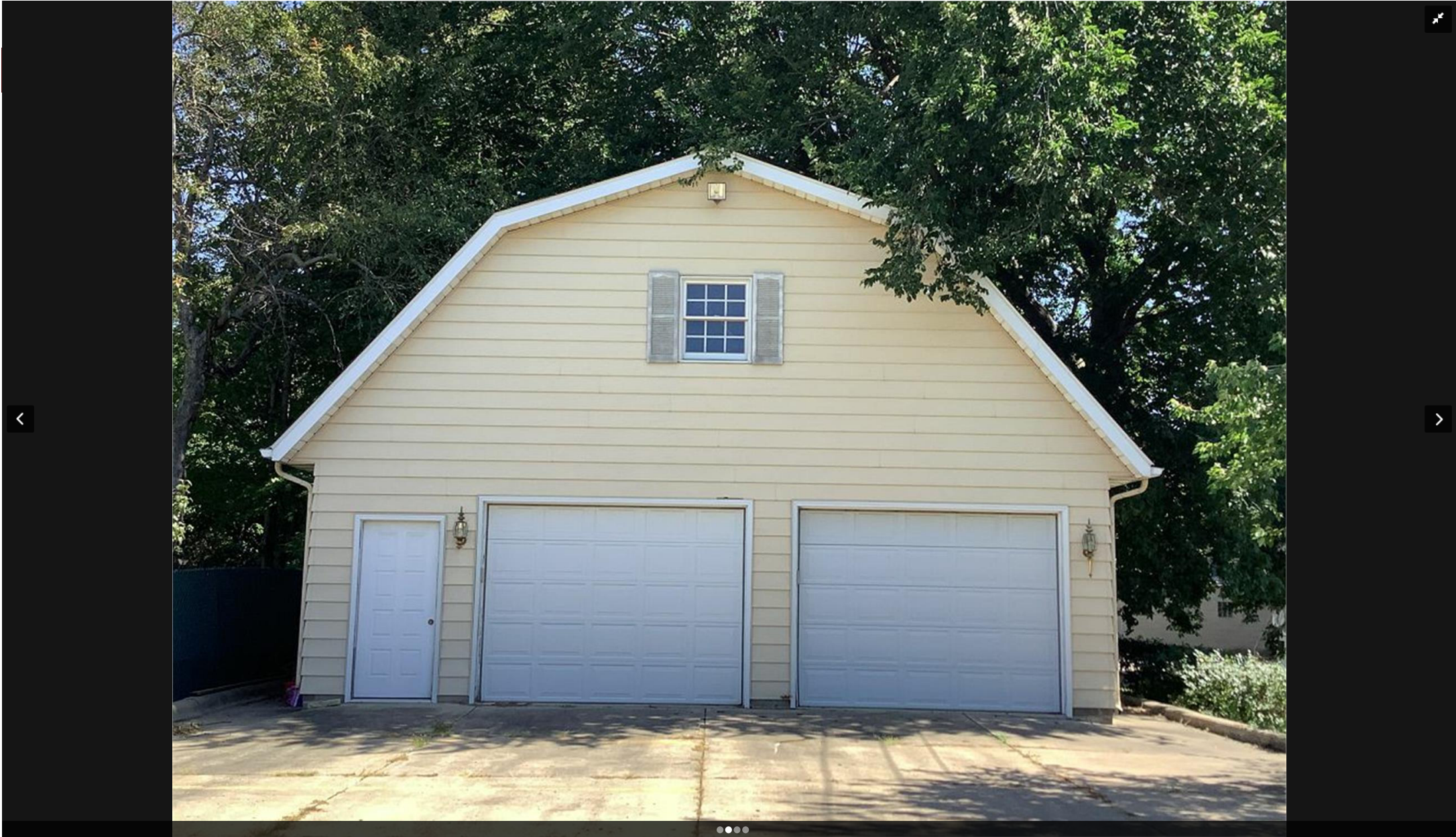
THE BEAST – AKA THE STRUCTURE TO BE RELOCATED
