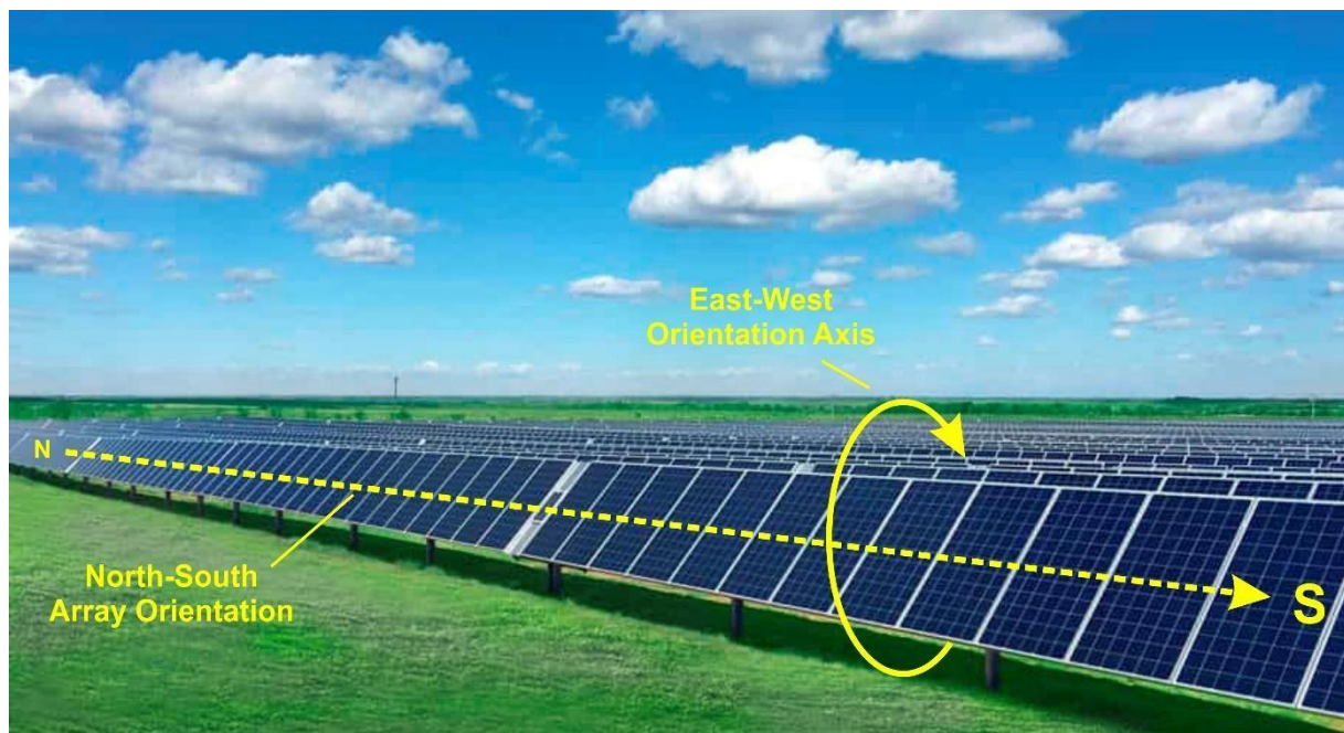
Figure 8: Diagram Showing Tracker Array Rotation and Orientation for the Proposed Project
