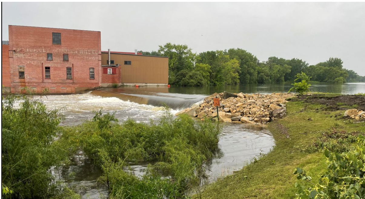
Photograph 5 South Dam Conditions after the Repair
