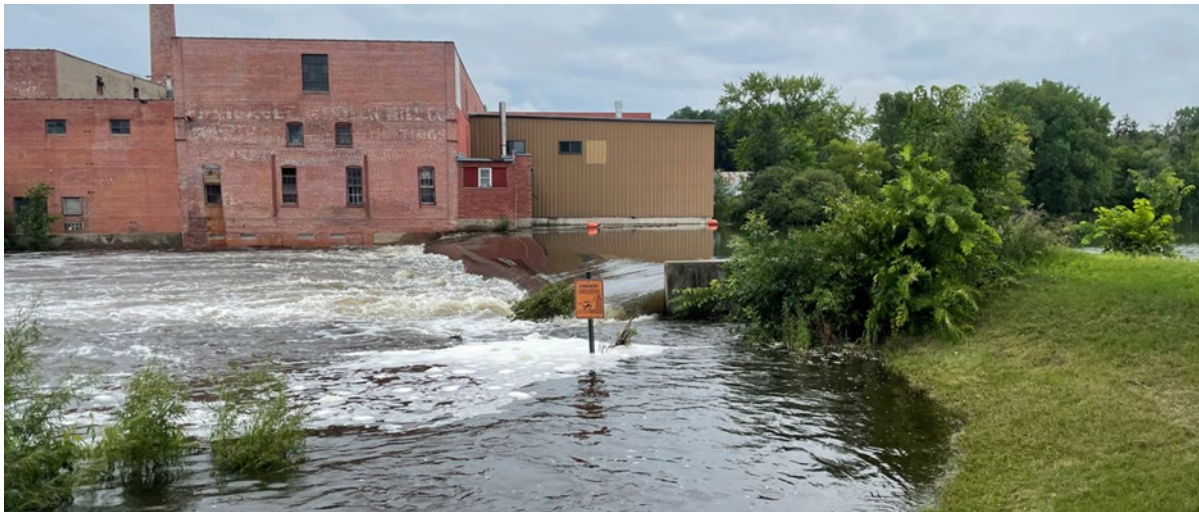
Photograph 1 South Dam on June 23, 2024
