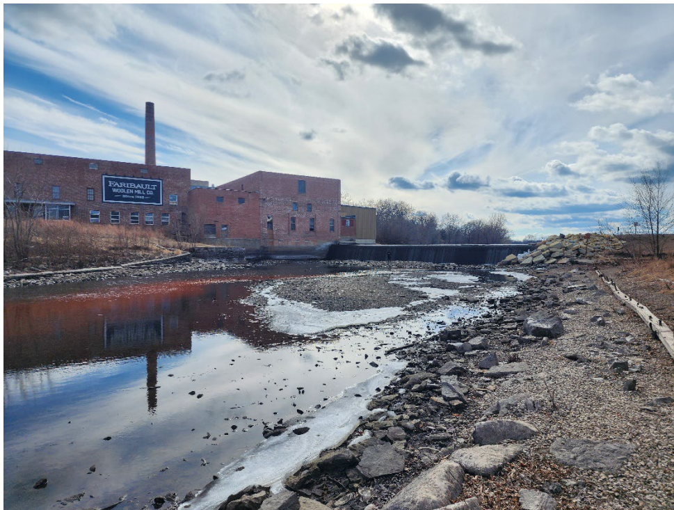
Photograph 1 Overall view looking Upstream at the South Dam
