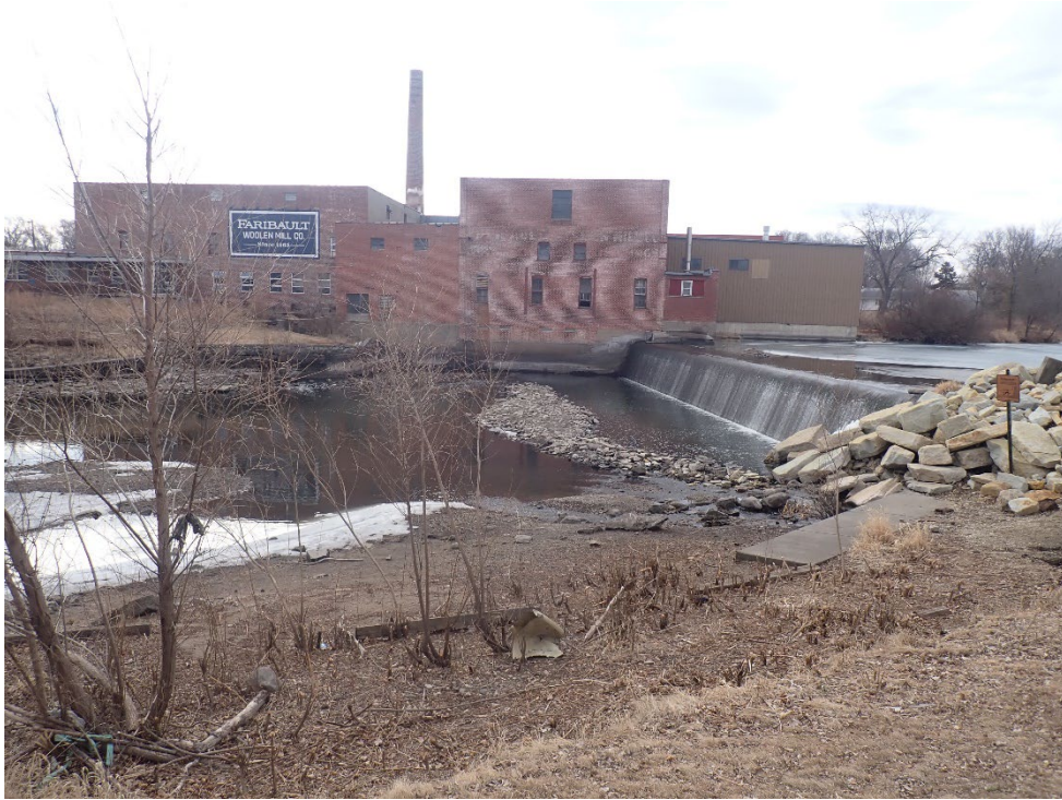
Photograph 2 Overall view of the South Dam looking right
