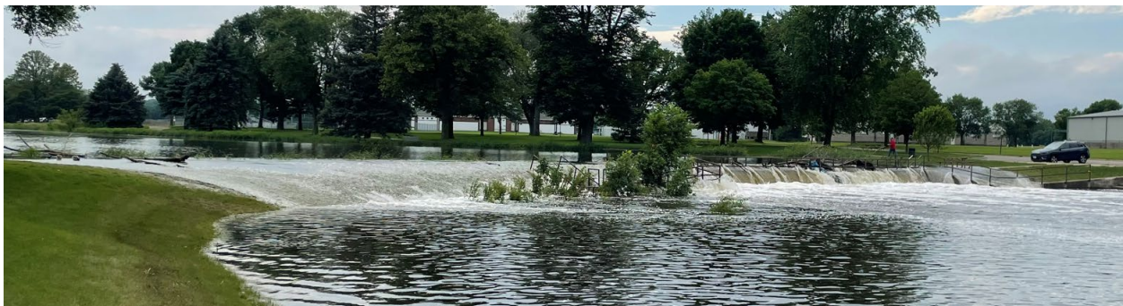
Photograph 3 South Dam on June 28, 2024
