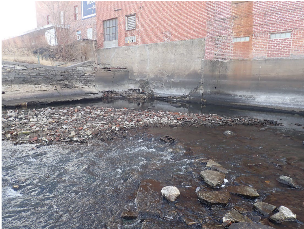
Photograph 13 Drains on the River Side of the Exterior Mill Building Walls
