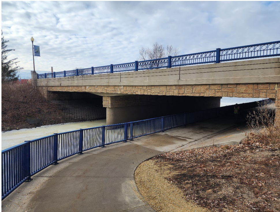
Photograph 16 2nd Ave Bridge Looking Upstream at the North Dam
