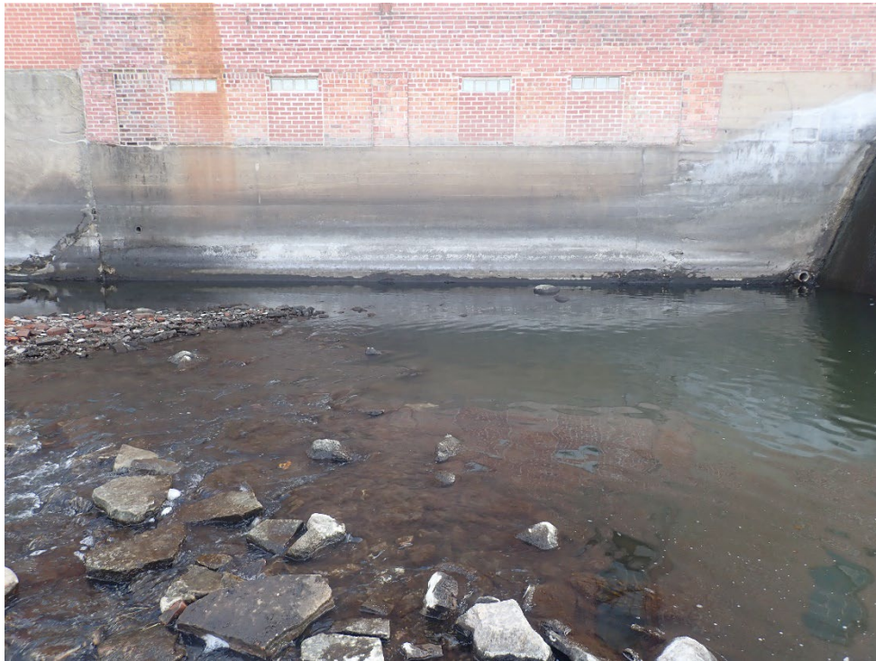
Photograph 12 Drains on the River Side of the Exterior Mill Building Walls
