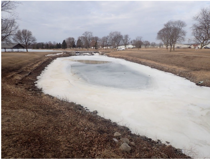
Photograph 14 Overall View Looking Upstream at the North Dam
