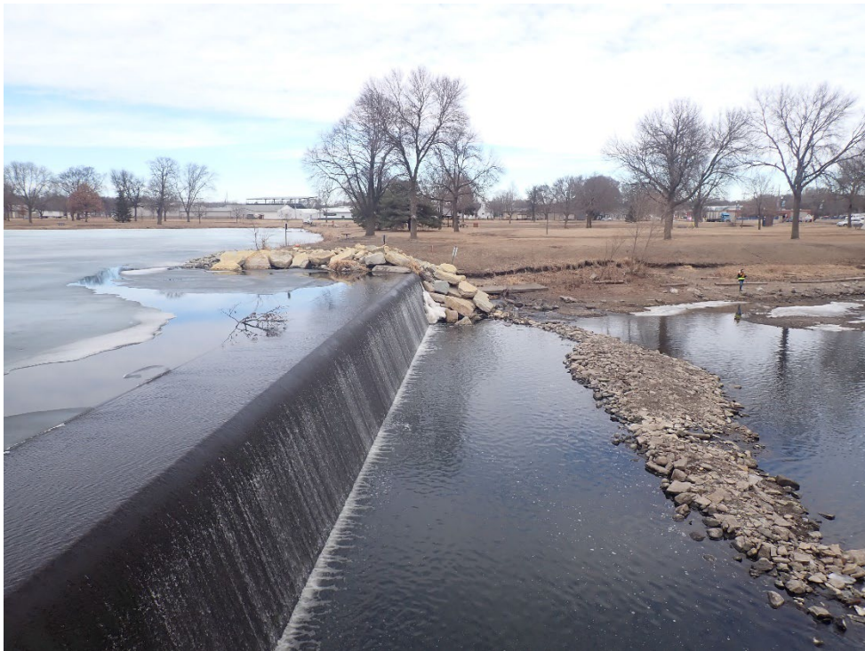
Photograph 3 Overall view of the South Dam looking left
