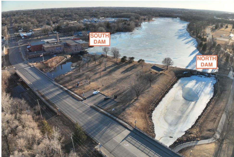
Figure 1 Woolen Mill Dam Naming Convention
