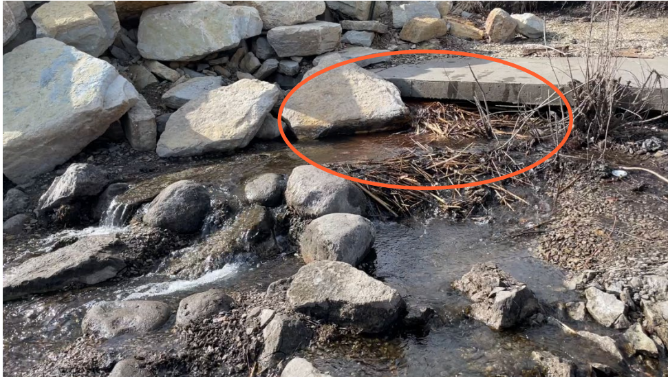
Photograph 10 Red Dye First Starting to Exit Downstream of the Left Abutment
