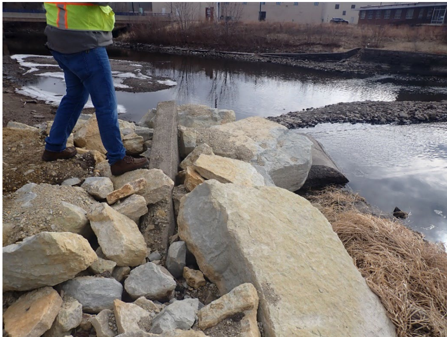
Photograph 7 Left Abutment Wall and Rock Repair
