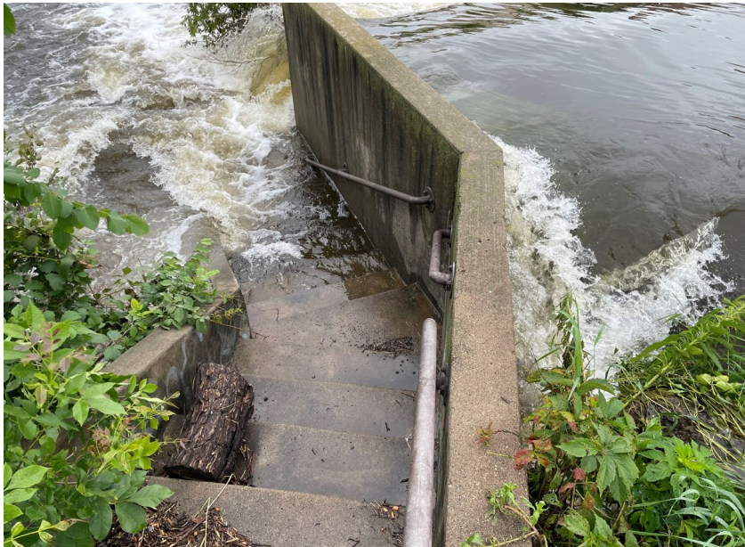
Photograph 2 South Dam on July 2, 2024
