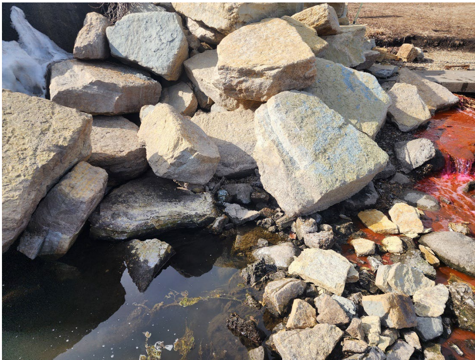
Photograph 11 Red Dye Traveling through the Left Abutment
