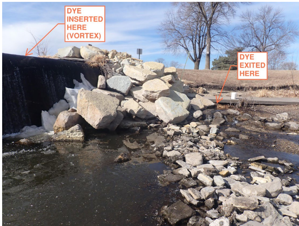
Photograph 9 Left Abutment Dye Test Setup
