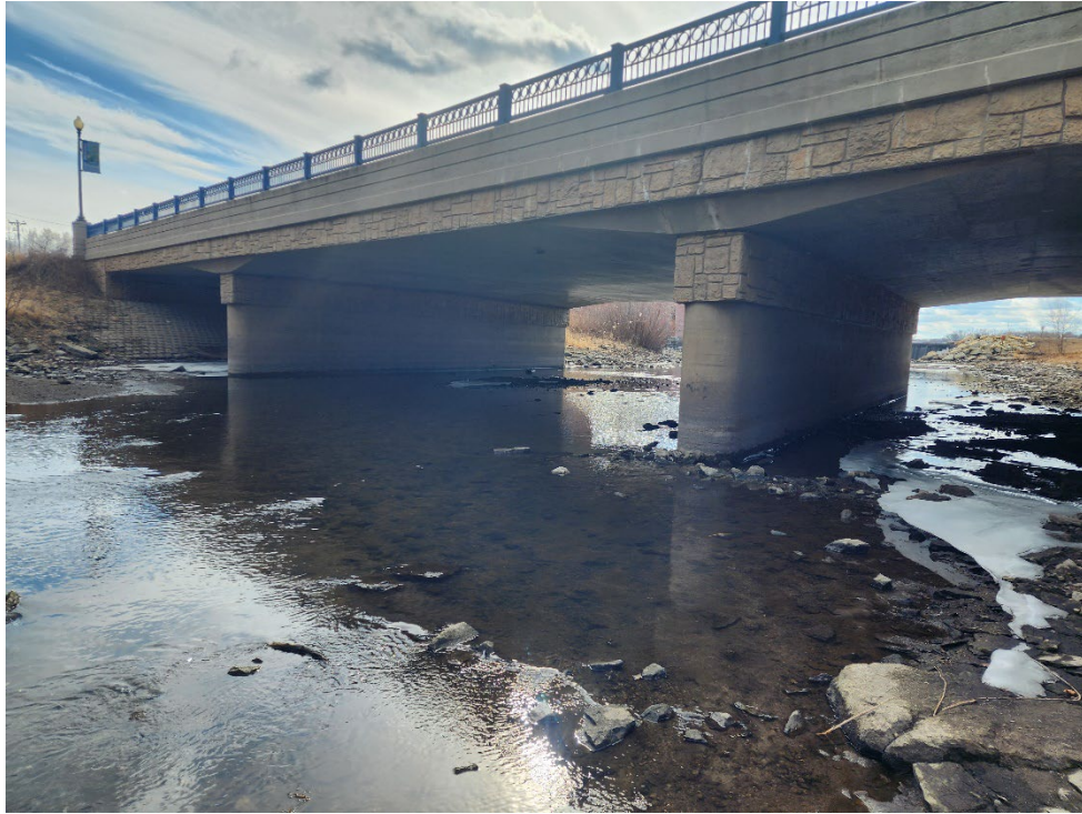
Photograph 5 2nd Ave Bridge looking Upstream at the South Dam
